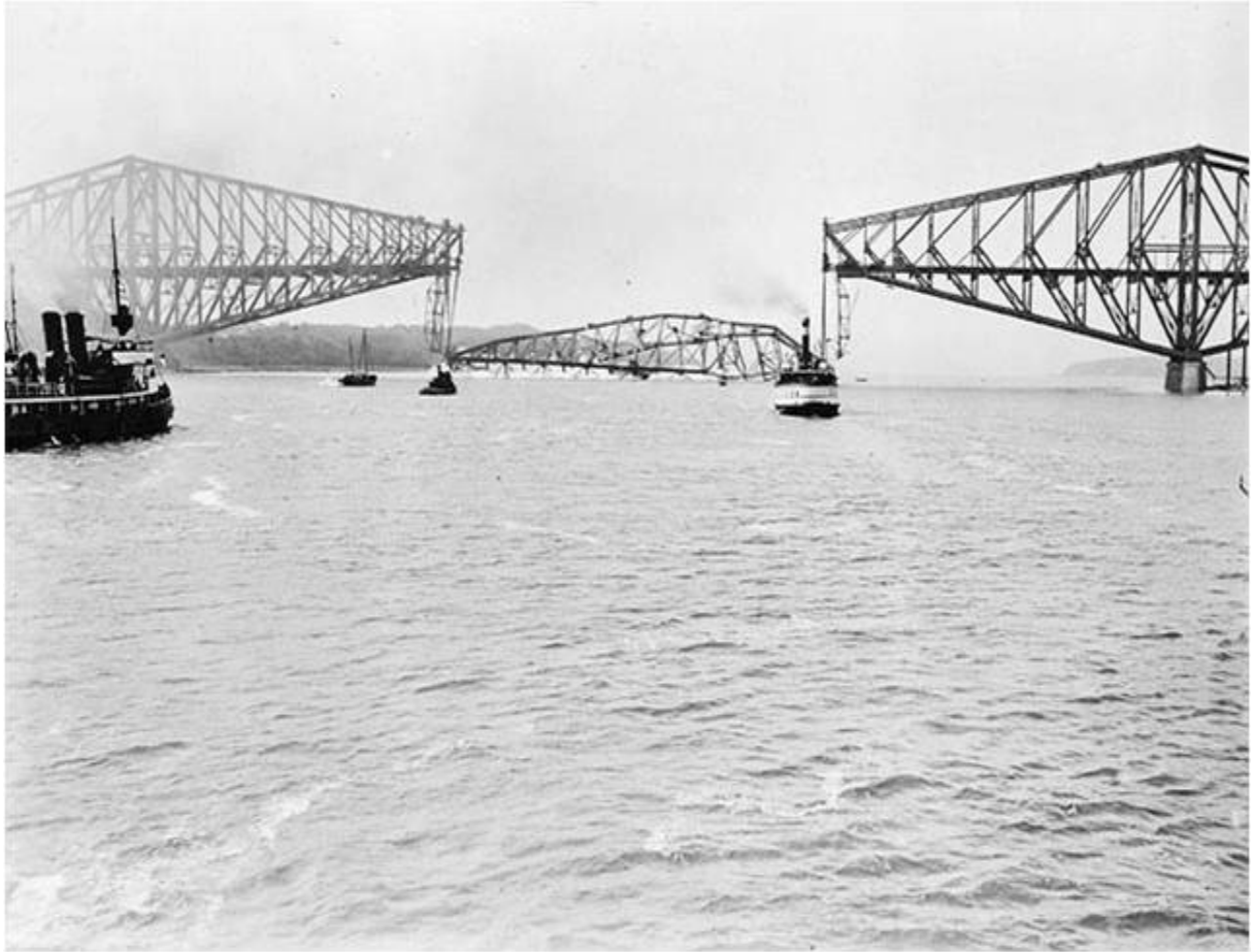
The Quebec Bridge collapsed on 11 September 1916 a second time due to poor design work and materials, killing thirteen workers. The bridge, which was conceived to be one of the most advanced in the world, had already collapsed under similar circumstances in 1907. In that tragedy, eighty-five workers perished prompting a Dominion Royal Commission to investigate the catastrophic failure.
