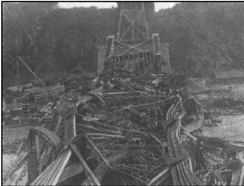
The twisted wreckage of the 1907 bridge. Image credit: Unknown author – Holgate, Henry; Derry, John, G. G.; Galbraith, John. (1908). Royal Commission Quebec Bridge Inquiry Report. Sessional Paper No 154. S.E. Dawson printer to the King Ottawa. Appendix 19, figure 20 ; scan found at http://matdl.org/failurecases/Bridge_Collapse_Cases/Quebec_Bridge
