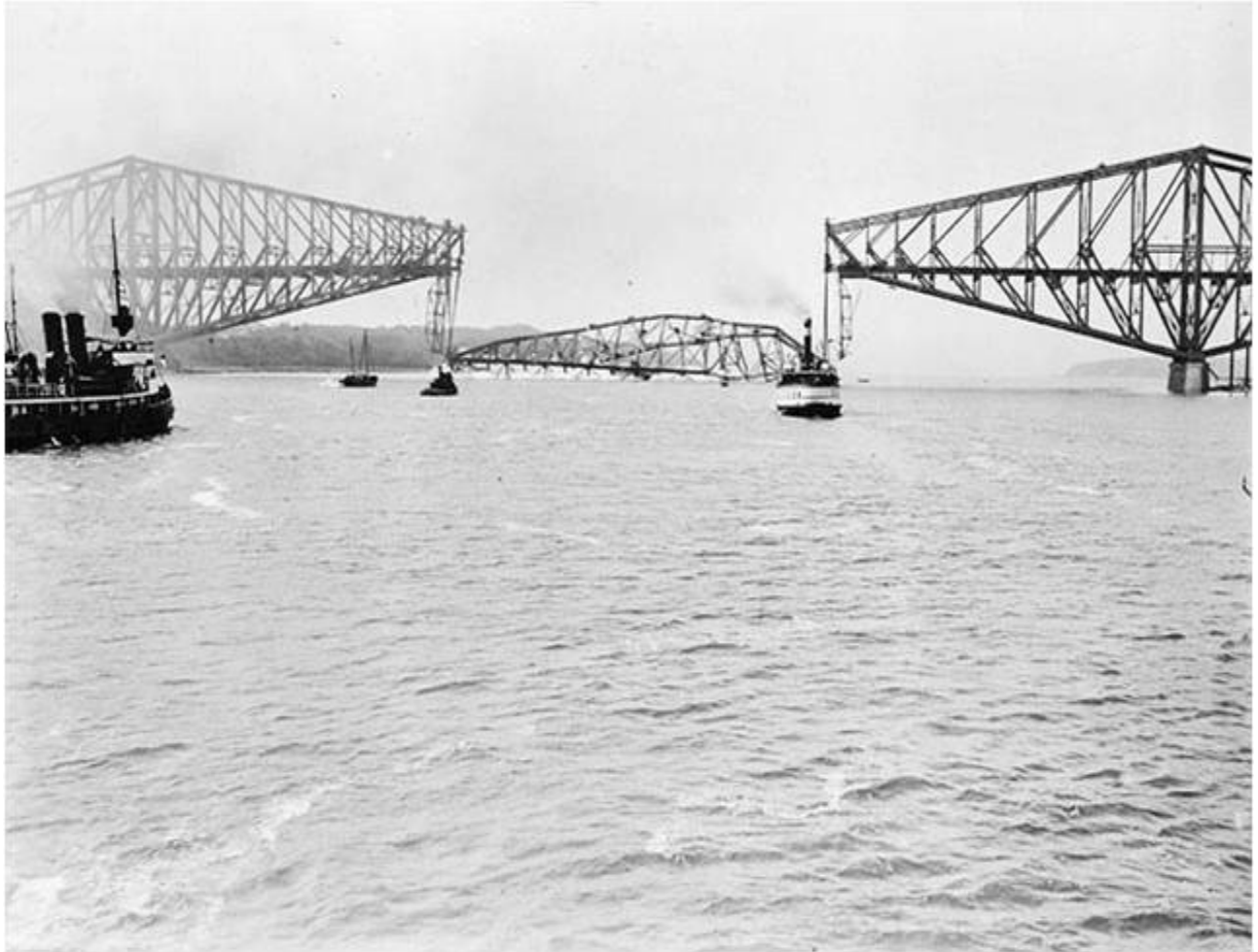
The Quebec Bridge collapsed on 11 September 1916 a second time due to poor design work and materials, killing thirteen workers. The bridge, which was conceived to be one of the most advanced in the world, had already collapsed under similar circumstances in 1907. In that tragedy, eighty-five workers perished prompting a Dominion Royal Commission to investigate the catastrophic failure.
