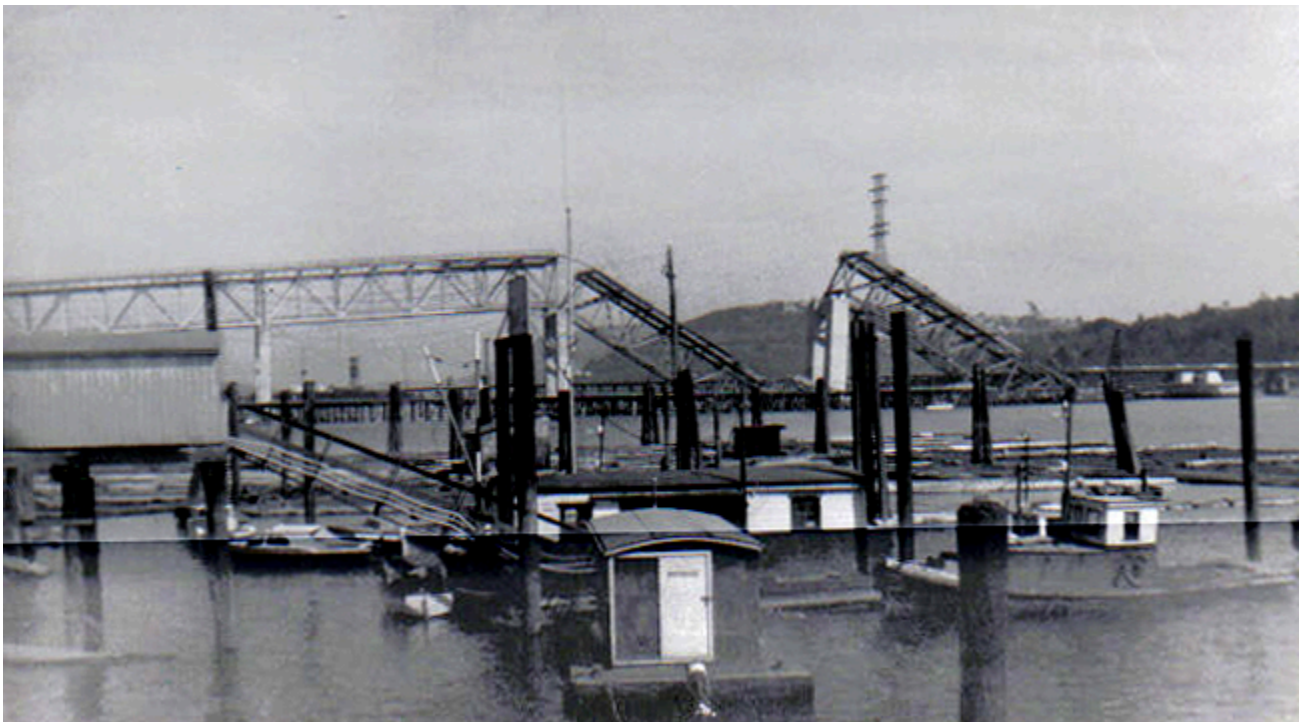
View (looking east) of new Second Narrows Bridge, 2 months after the collapse of 2 spans, Image credit: Ron Thomson, Personal Collection CC BY-SA 3.0 File:Second Narrows Bridge (Vancouver).jpg Created: 17 August 1958
