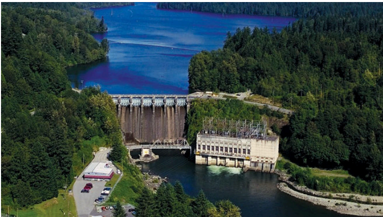
Figure 1. Ruskin Dam on Hayward Lake near Mission BC. Source: BC Hydro
