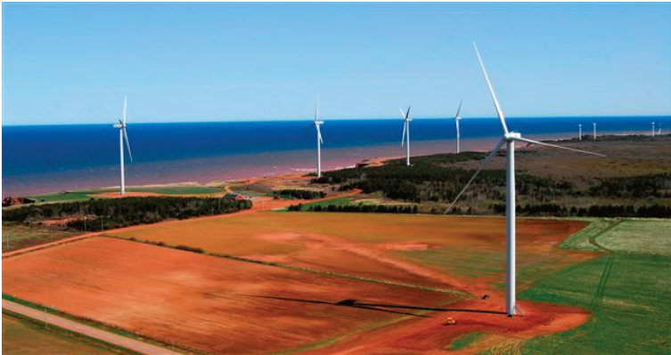
A research and development wind farm, operated by the Wind Energy Institute of Canada in PEI. Source: Natural Resources Canada
