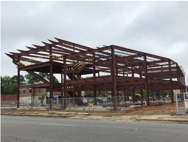
Non-Insulated Steel Beam
