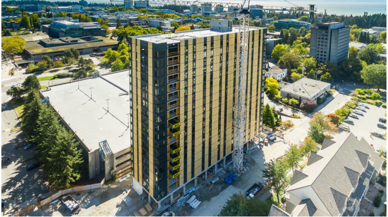
Figure 23. An 18-story hybrid mass timber residence at the University of British Columbia (UBC). Source: http://news.ubc.ca .
