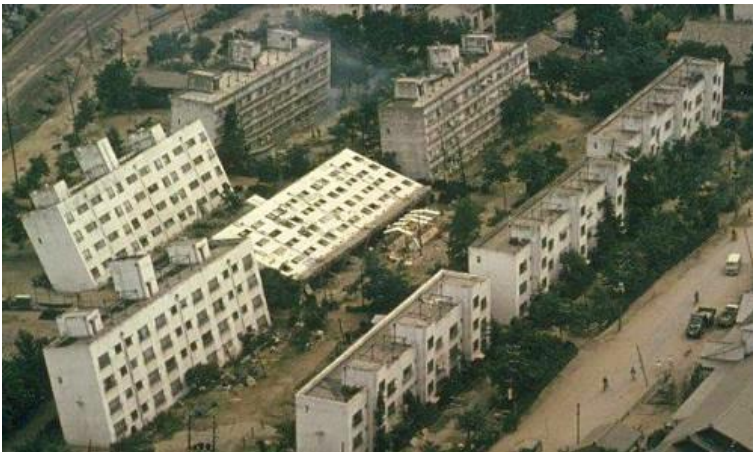
Figure 11.22 Collapsed apartment buildings in the Niigata area of Japan. The material beneath the buildings was liquefied to varying degrees by the 1964 earthquake. http://en.wikipedia.org/wiki/1964_Niigata_earthquake#/media/File:1964_Niigata_earthquake#/media/File:Liquefaction_at_Niigata.JPG
