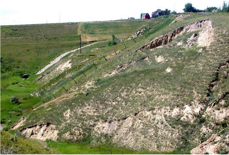
Figure 15.15 A slump along the banks of a small coulee near Lethbridge, Alberta. The main head-scarp is clearly visible at the top, and a second smaller one is visible about one-quarter of the way down. The toe of the slump is being eroded by the seasonal stream that created the coulee. [SE 2005]
